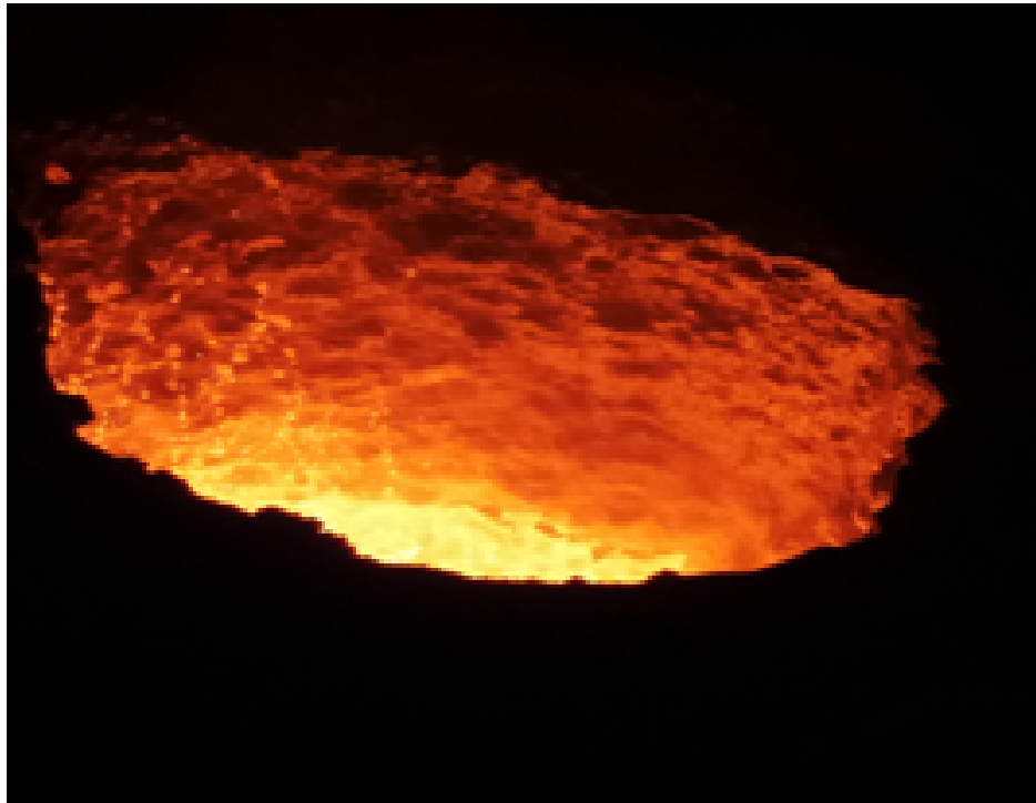
Furnace Condition Before
