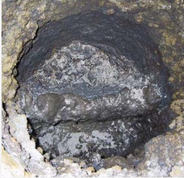
Closeup of Pocket before Redux treatment
